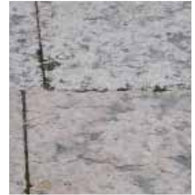
lastre in pietra locale
